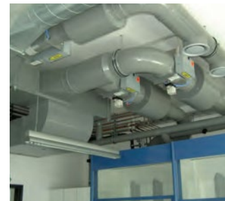
Fume vents, ducting: SIMONA® PVC Type I
